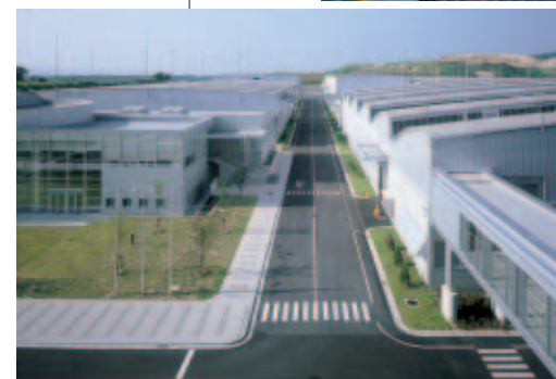
Road on the east side of the Kyotanabe Plant
