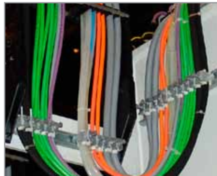
B Saddle style - Screw-down modular clamps C Block style - Screw-down split block clamps
